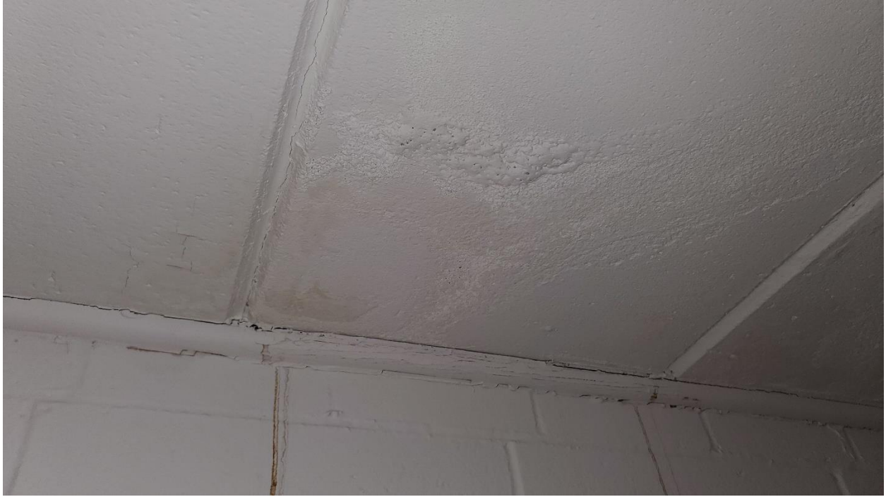
Figure 5: 1963 Addition - Evidence of water infiltration at northeast corner.
