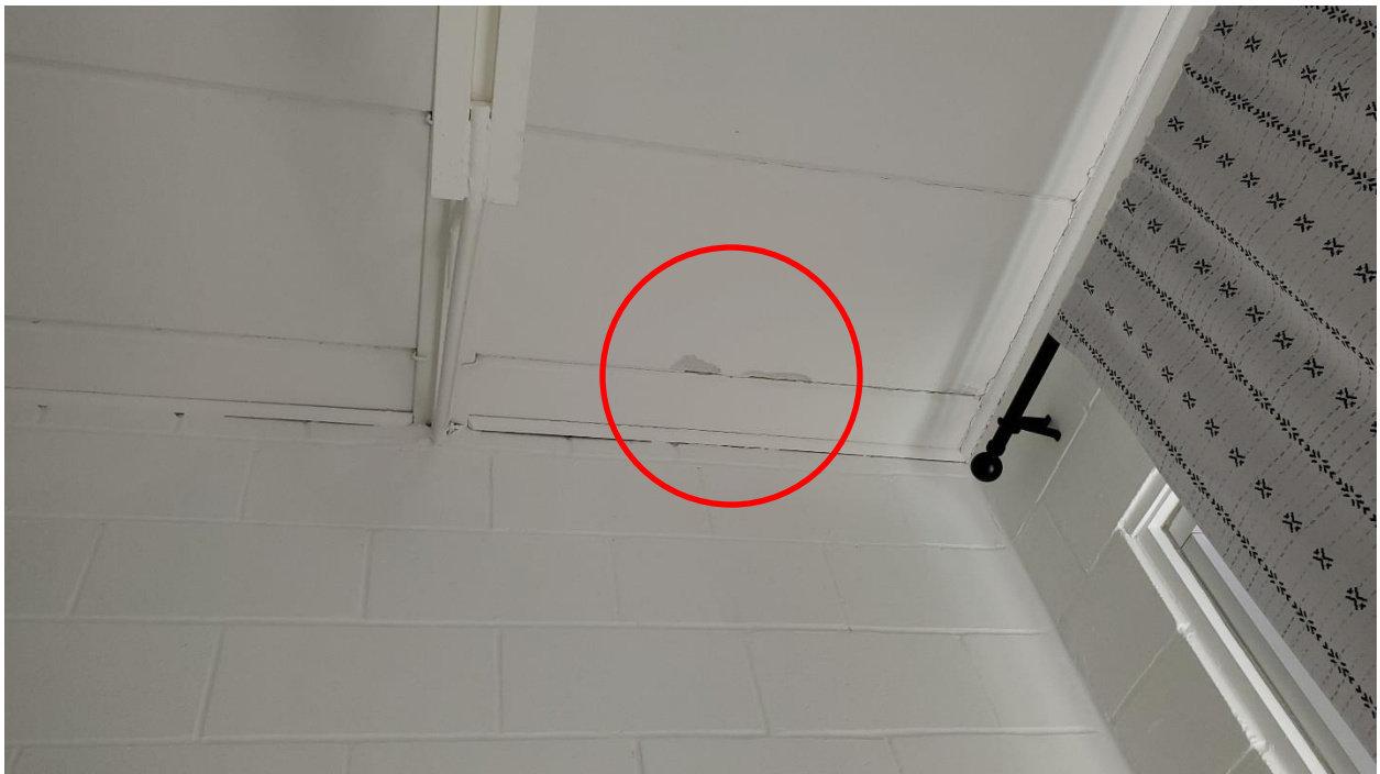
Figure 6: 1963 Addition – Minor surface damage to a slab at the southeast corner.
