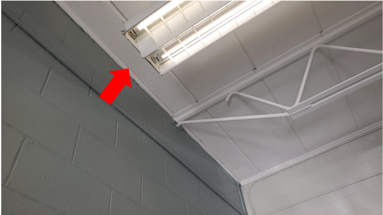
Figure 7: 1963 Addition – Evidence of water infiltration at the southwest corner.
