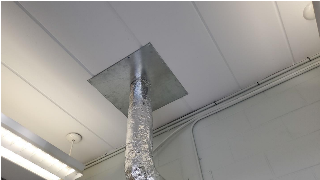
Figure 8: 1963 Addition – Mechanical penetration through Siporex slabs.
