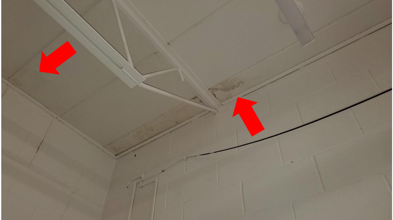
Figure 3: 1963 Addition – Evidence of water infiltration at northeast corner.
