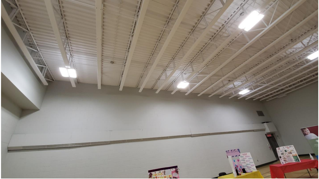
Figure 9: 1973 Addition - Typical high roof framing.
