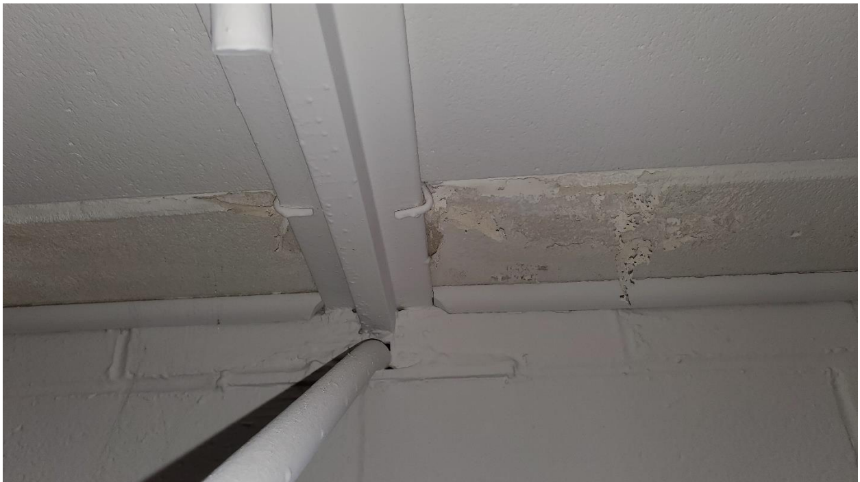
Figure 4: 1963 Addition - Evidence of water infiltration at northeast corner.
