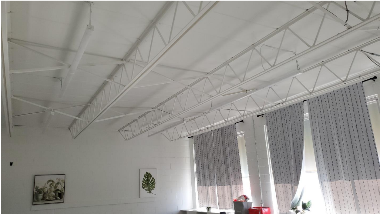
Figure 1: 1963 Addition - Typical roof framing over classrooms.
